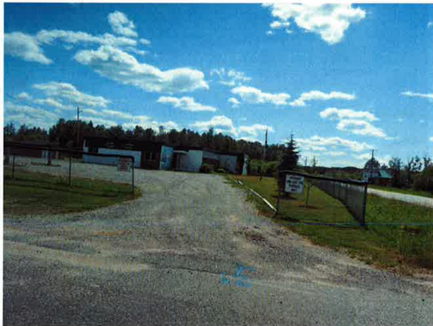
ENTRANCE FROM SHERRY AVE.
